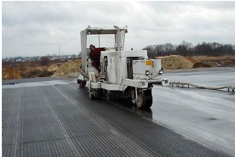
Figure A6-5. Grooving with saws
